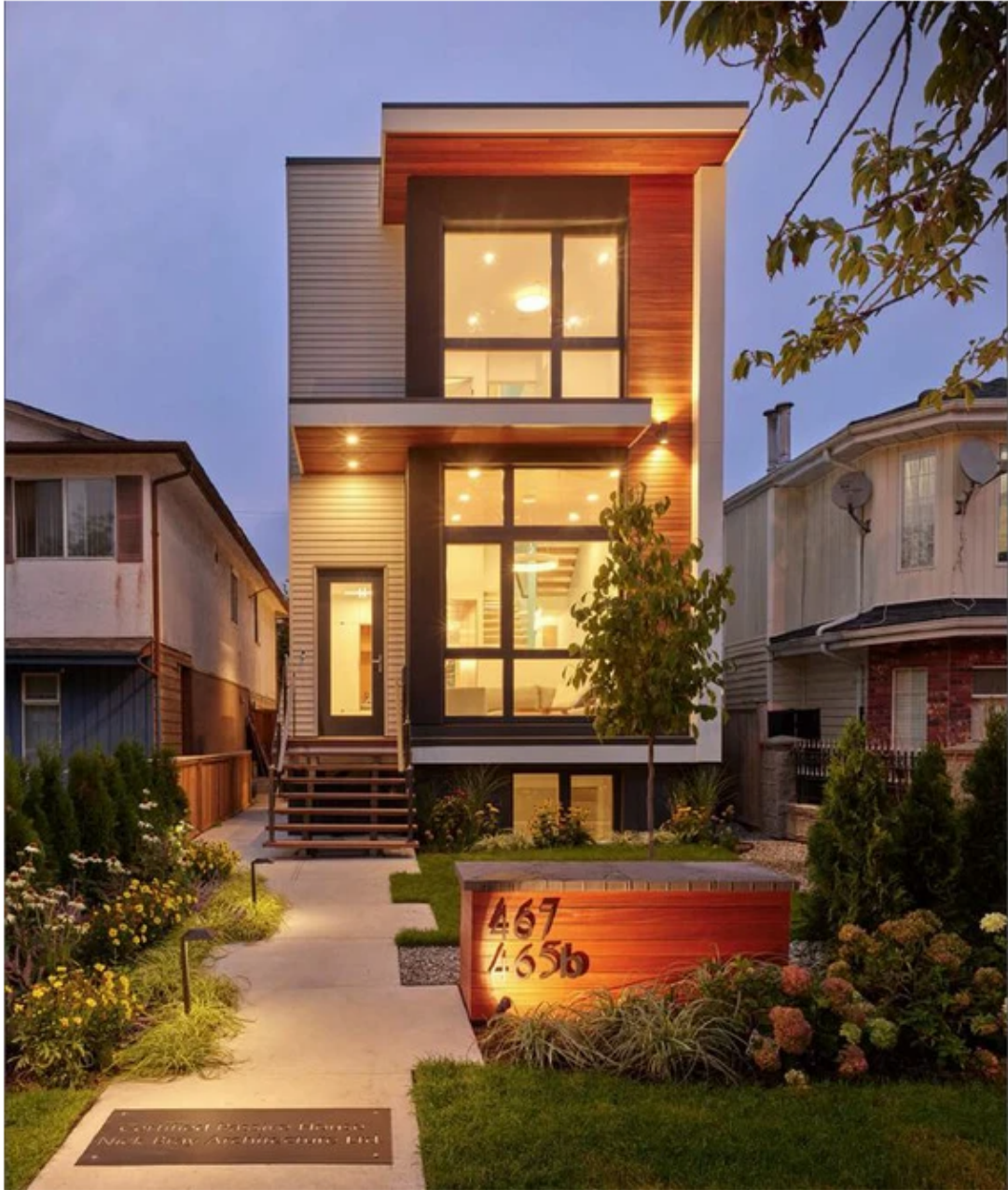
Nick Bray designed the "Passive Narrowtative" house to make the most of a skinny urban lot in East Vancouver. PHOTO BY SUPPLIED /PNG
